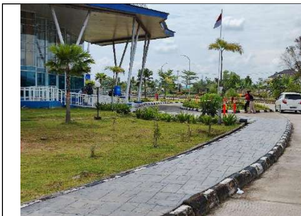
A safe and comfortable road for pedestrians
