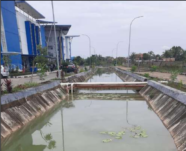
Water Conservation – Canals (UIN Raden Fatah Palembang, Indonesia)
